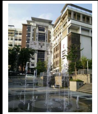
KUALA LUMPUR HOSPITAL, MALAYSIA
